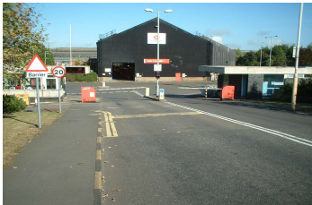
Site entrance, put on all PPE
