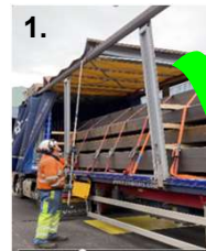
1. Close roof from ground
