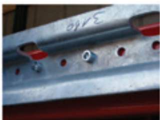
Figure 11: Anchorage bar
