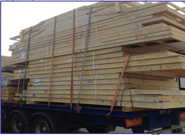
External wall panels on bottom, internal on top
