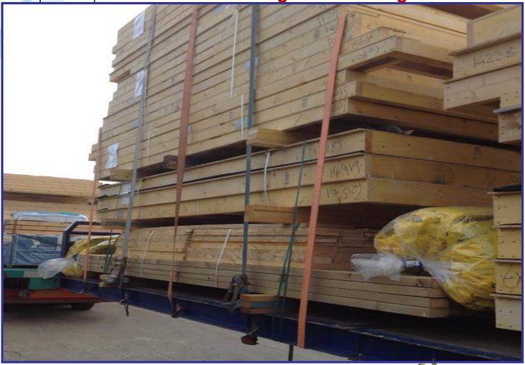
Mixed load of External wall panels, Loose material and internal wall panels
