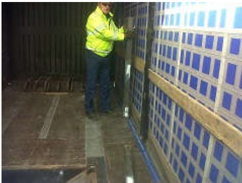
4. Prepare trailer bed
