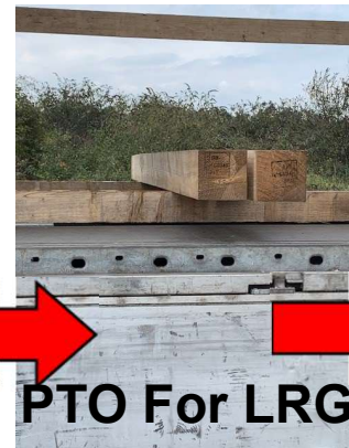
Get 8 X Anti-slip Matting Place under base timbers (on top ALSO in Winter Weather Period)
